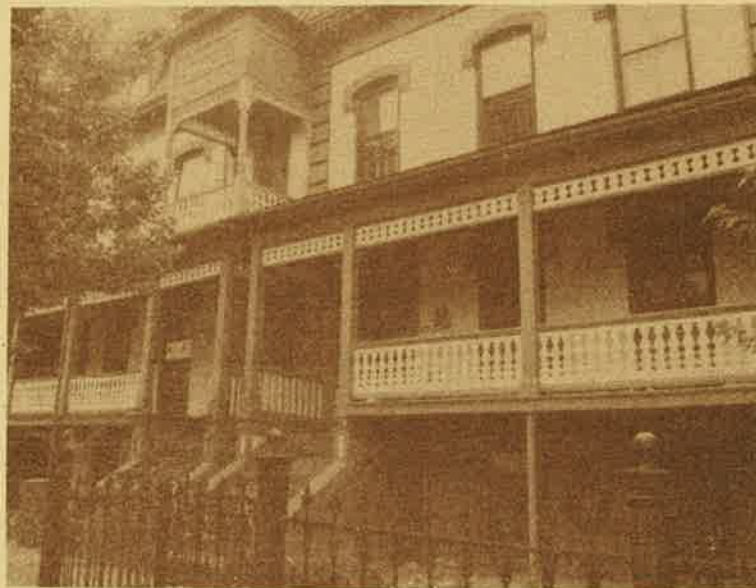
Elegant 1860's brick rowhouse, first of a series of complexes which transformed the Mattoon Street District into the only complete rowhouse neighborhood in Springfield. This Second French Empire residence had lain vacant for twenty years before its renovation in 1977.
