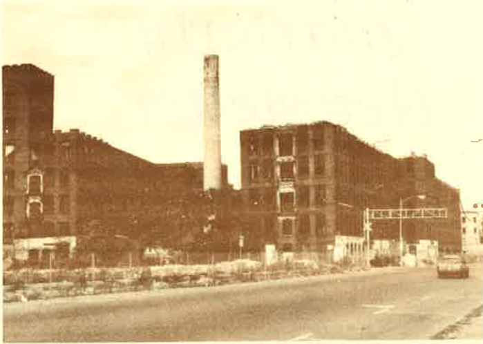
Indian Motorcycle Building before renovation. The smoke stack is no longer there, but the other buildings are intact.
