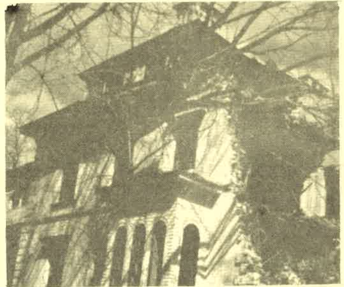
Tiffany-Bowles House in the process of being demolished.
