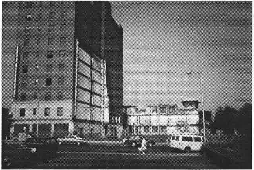
Charles Hotel days before demolition
