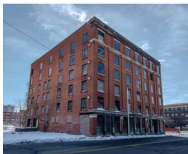
The now-vacant building has been in municipal possession through tax-foreclosure since September 2009. Over those nearly eight years, no steps have been taken to secure the structure from water penetration. No inspection was made following the 2012 Gas Blast, which occurred 425 feet away, to determine damage
