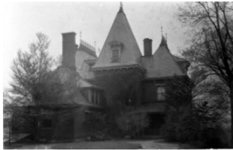
Photo Courtesy of Works Progress Administration, 1939
