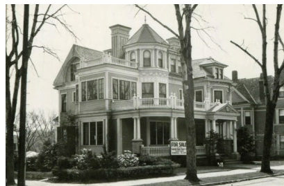
Image by Public Works Administration, 1939
