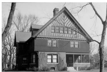
Image by Public Works Administration, 1939
